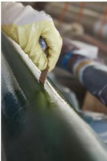
The execution of the repair work is closely inspected for quality.
