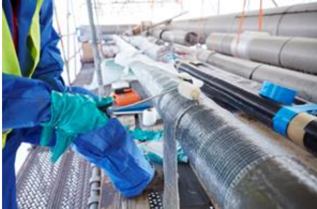
Application of the first layer of Loctite PC 5085 glass-carbon fiber tape.
