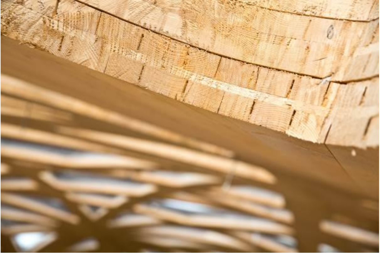
Glulam timbers for the roof, cross-laminated with Loctite Purbond.
